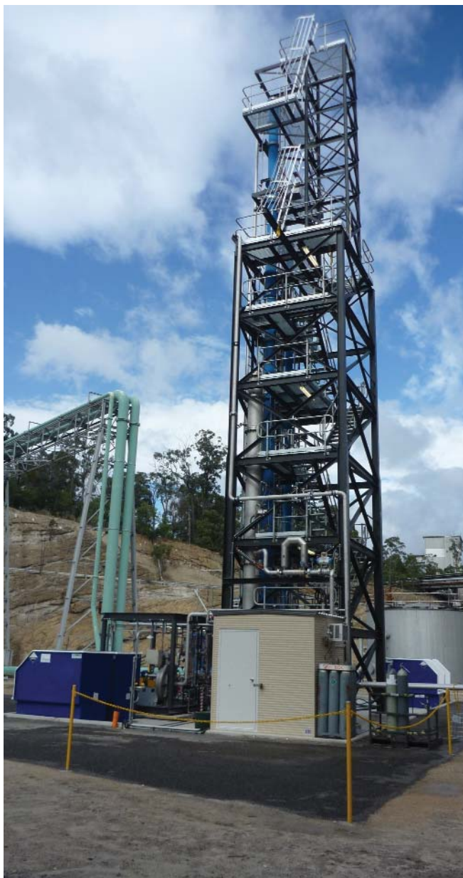
The PCC pilot plant at Tarong Power Station is designed to capture approximately 1000 tonnes of CO 2 per year (Image: CSIRO)
